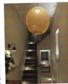
LED lights on a motion sensor save energy. It's a great option for bathrooms and staircases, as in this scheme by John Cullen Lighting ( www.johncullenlighting.com )
